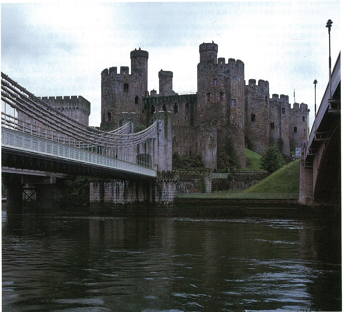
Conwy Suspension Bridges, Wales
